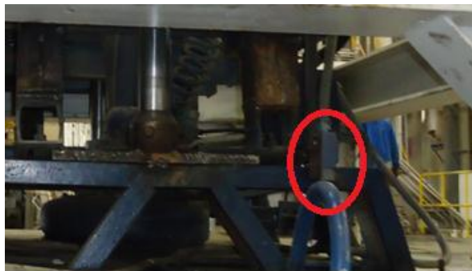
Fig. III.67. Sensor cilindro molde sube
